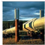
Trans Alaska Pipeline
